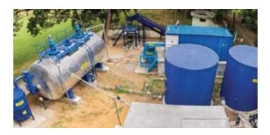
Pilot Plant at CSIR-CLRI, Chennai for co-digestion of vegetable market waste and slaughterhouse waste using bioextruder as pre-treatment. This can be used as a demonstration model plant in the waste management of smart cities.
