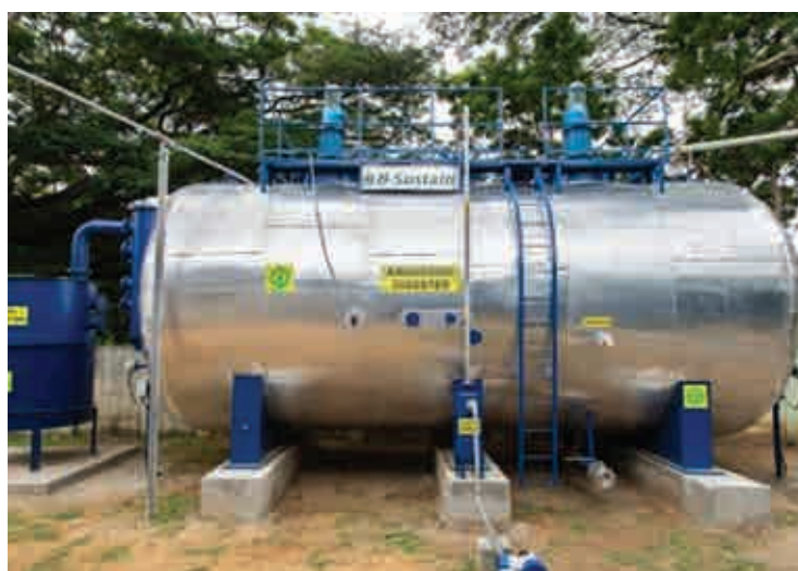
Digester with top mounted twin agitator
